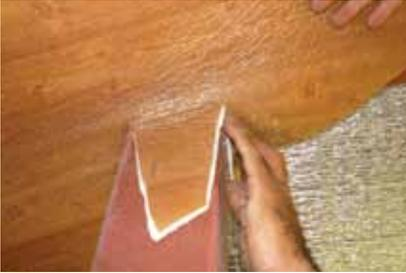
5.1 In case there are two columns in the place where the structure will be placed, cut and try to obtain the same shape as that of the PRODEX Rustic®.
