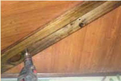
6.2 Screw the 2" wood piece on the frame skeleton by covering the fastening pieces and the joints of the rolls of PRODEX Rustic®, using a 2" fine tip screw.
