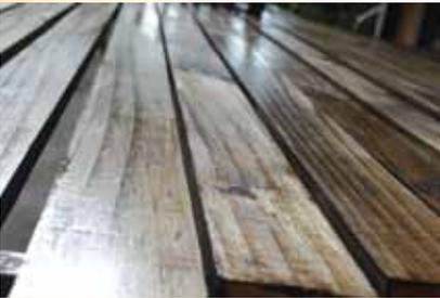
1.2 Choose and prepare wood of 2" wide and ½" thick; these pieces will be used later on the beams during installation. Consider an amount of 80 linear meters of board per each 100 square meters of ceiling and using pine, laurel, teak, or your choice of wood. To get a better finish, you can dye or varnish the piece as you wish.
