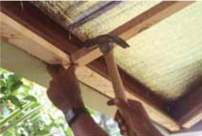
2.2 Assemble the boards with 1 ½" nails; use a 1 ½" drill tip to fasten to the cold rolled C section, if necessary.
