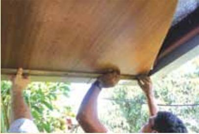
4.1 Once the PRODEX Rustic® is placed, fasten it to the frame skeleton by placing a fourth round board on top so that the board acts as a support and pressing at the same time; therefore, you can handle the PRODEX Rustic® and get the required position.
