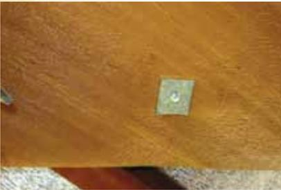
4.2 Use the head screws for the ceilings or build small 1" x 1" tin squares to fasten the insulation to the wood of the frame skeleton across the structure. Remember that you will have flexibility with the placement of the PRODEX Rustic® so that you can get the proper position thanks to the over measurement of the initial cutting.
