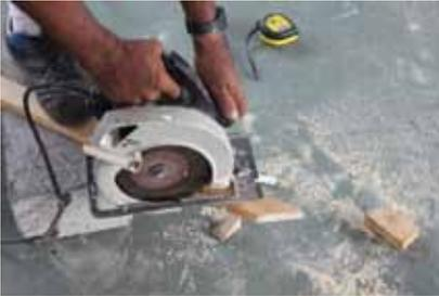
2.1 With 1 ½" x ½" wood board, make a frame skeleton with a configuration of 1.20 meters of distance between boards; these will be the points where the rolls of Prodex Rustic® will be installed.
