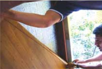
5.2 With the line drawer, draw a mark in the middle of the wood beam to which the Prodex Rustic® was fastened.
