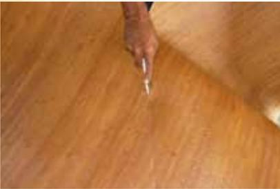
3.2 Carefully cut the Prodex Rustic® with a blade by following the drawing.
