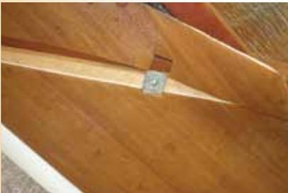
5.3 Remove the excess PRODEX Rustic®, this is the over measurement left at the beginning of the installation.
