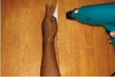
6.1 PRODEX Rustic® has a 3 mm thermo-welded platform to join the overlaps of two rolls, if necessary. This process is carried out by applying heat to the edges of the foam that are exposed and pressing a little with the palm of your hand; with this type of joint, the completely impermeable mechanical seal is guaranteed between both rolls.
